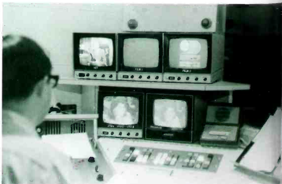
Fig. 1 At WESH-TV, the problem of lack of space for picture monitors was solved by the monitor-stretcher in operation here. See schematic in Figure 2.
